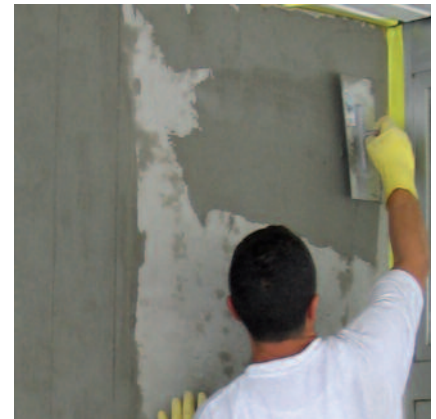
PCI Barrafill L for cosmetic work on concrete components.
