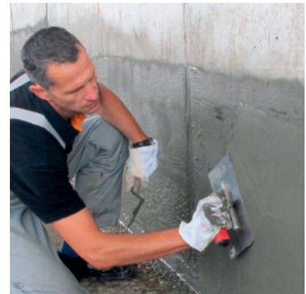
PCI Barraseal is creamy and workable, pores and cavities can be closed easily and rapidly.
