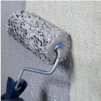
Apply a contact layer using a roller.
