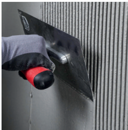
The last applied layer is smoothed to produce a smooth, fine textured surface.
