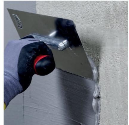
A contact layer can also be applied as a scratch coat.
