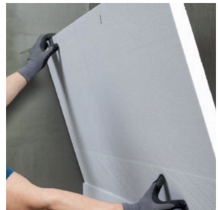
PCI Barraseal Turbo is used to glue drainage boards and insulation boards to the substrate.
