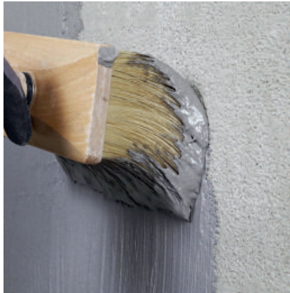
Apply a contact layer using a brush or flat bristle brush.
