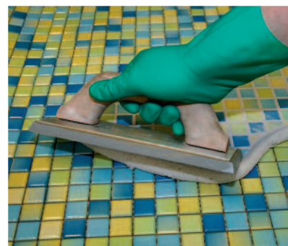
Chemical resistant and water impermeable grouting of mosaic coverings with PCI Durapox NT and PCI Durapox NT plus.
