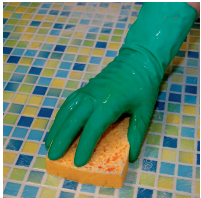
Washing the grouted coverings with the soft PCI epoxy sponge.
