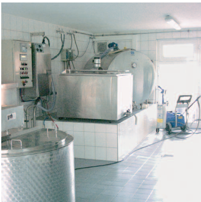
Highly wear resistant and chemical resistant laying and grouting of ceramic coverings, e.g. in dairies.
