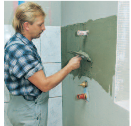
PCI FT Extra is non sagging, the bedded tiles immediately bond but can still be adjusted to correct position.
