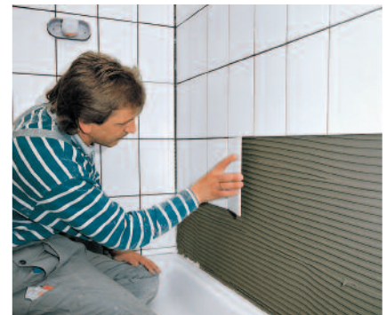
Reliable laying of non-vitrified tiles with PCI FT Extra on the waterproofing layer PCI Lastogum.
