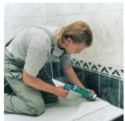
Corner joints, connection joints and movement joints are sealed with an elastic joint sealant.
