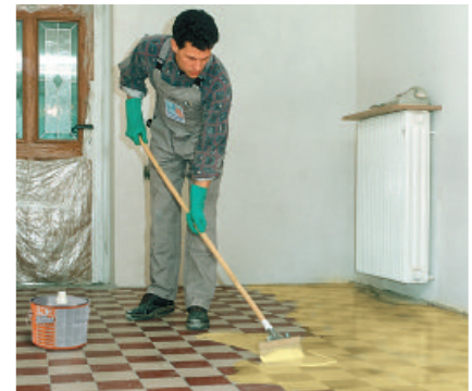
PCI Gisogrund 303 is the reliable primer for laying coverings on ceramic tiles and flagstones.
