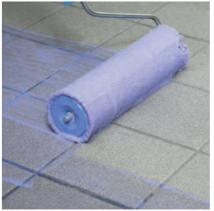
PCI Gisogrund 404 in violet dye enables a high bond strength of levellers and coverings to the respective substrate.
