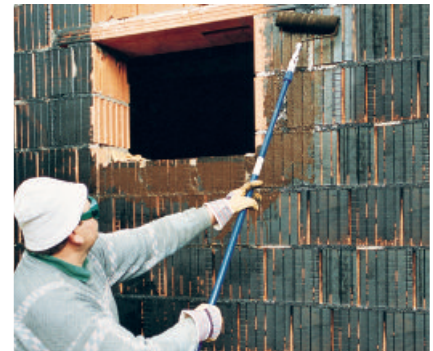
PCI Pecimor F, diluted 1 : 5 with water, acting as primer for waterproofing buildings with polymer-modified thick bitumen coating to DIN 18 195.
