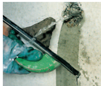
Water leaks can be quickly stopped with PCI Polyfix 30 Sek.
