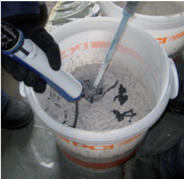
Add component B to the compound and remix for at least 2 minutes.
