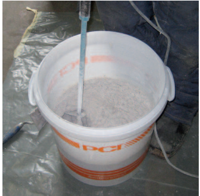
Mix for approx. 1 minute until compound is homogeneous and free of lumps.
