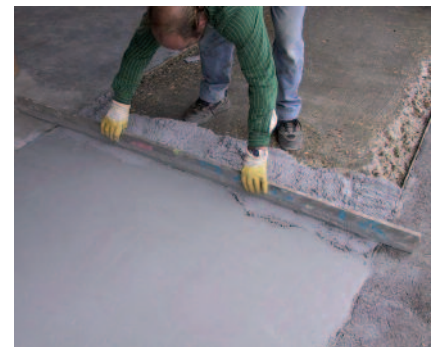
Surfaces subject to mechanical loads can be repaired - without priming - with PCI Repafast APS 40 down to -25 °C.
