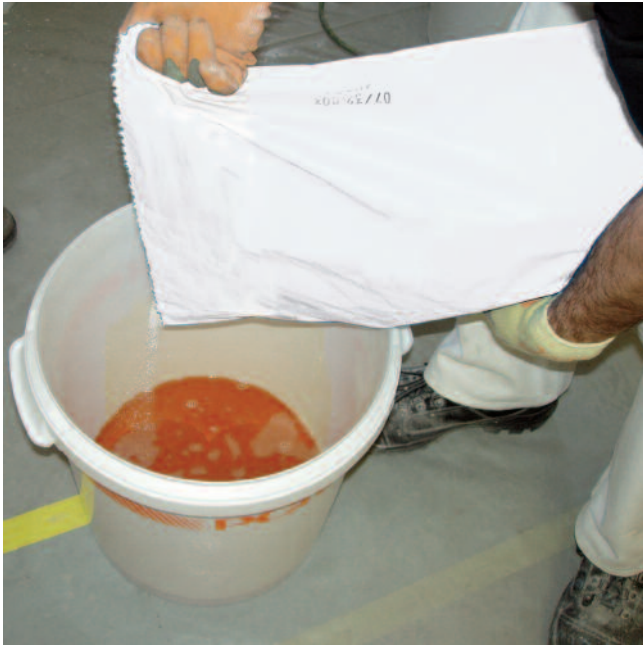
Pour content of component A in a blade-type mixer and add component C.
