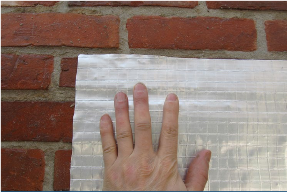
Press the Reaxyl® Benfoil 31 in the fresh Reaxyl® ZX-345 brick slip glue.
