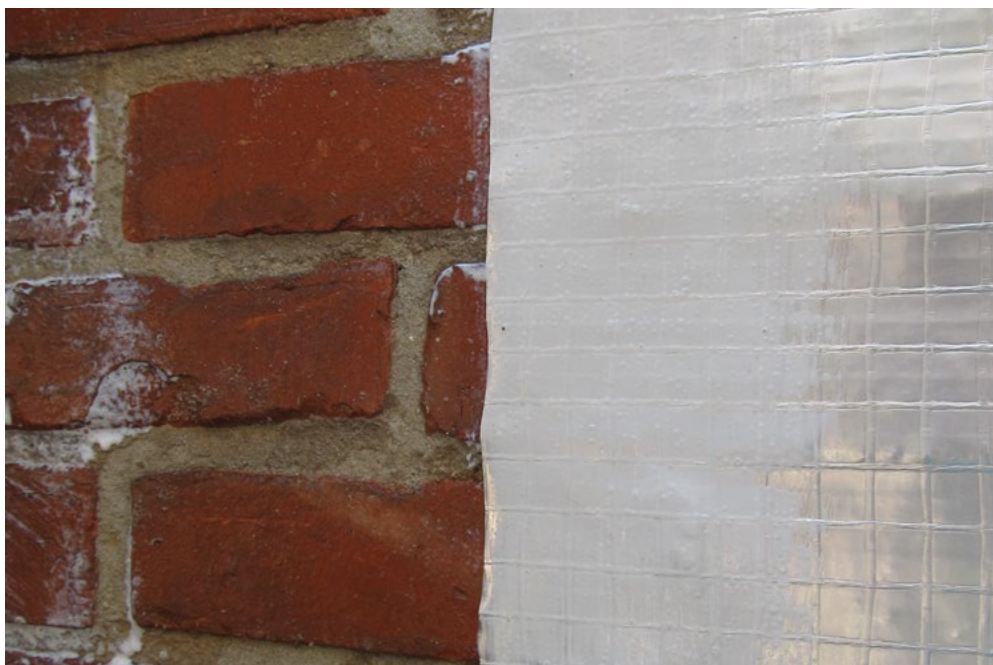
Overlap seams and joints 5 – 10 cm with Reaxyl® Foliad.
