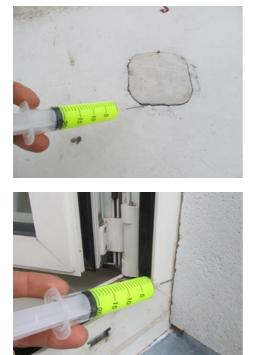
Apply the with water diluted fluorescent dye under the roofing with the help of the included dosing needle.
