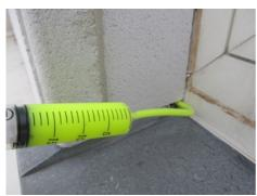
Apply the with water diluted fluorescent dye between fine gaps, in cracks or joints with the help of the included dosing hose.
