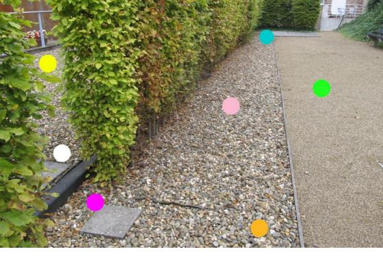
Colour division to search for leaks in roof gardens. Compartmentalize the roof garden into 7 colours. Do not forget to write this down.
