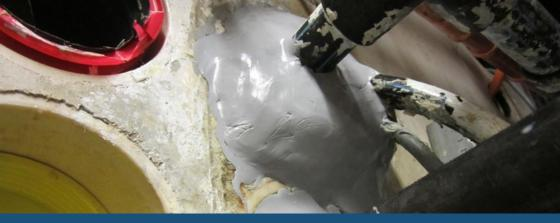
Reaxyl® Tubefix® is a sealant for waterproofing all ducts like gas, water, electricity, high voltage, cable-TV, telephone, fuel oil (mazout), etc. between the pre duct of the concrete and the drain(s) or cable(s). Tubefix has an exceptional adhesion, elasticity, temperature resistance and waterproofing up to -40°C / +95°C (30 min. to +155°C) and also resistant to vibrations and it is paintable over, silicone-free, mold and bacteria repellent, UV-resistant and durable.
