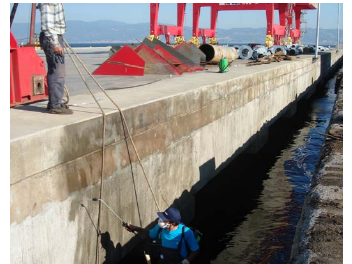
Yilport Jetty, Kocaeli, Turkey
