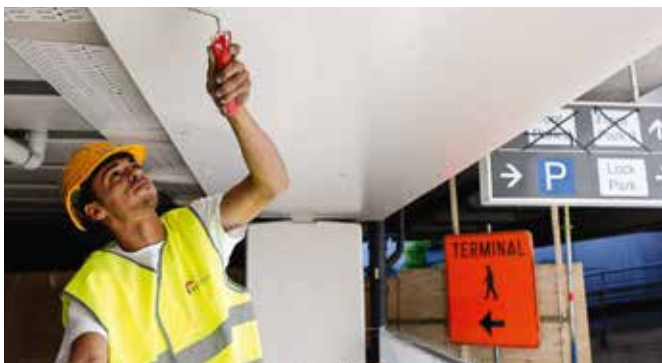
Manual Application of MasterProtect 330 EL (Carpark Airport Brussels, Belgium)
