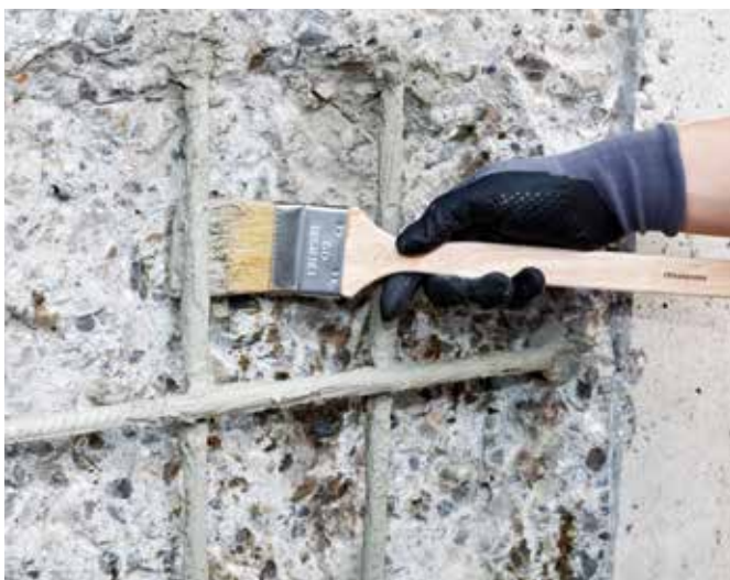
Application of MasterEmaco P 5000 AP on cleaned reinforcement
