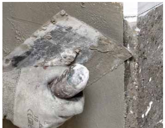
Levelling of surface with MasterEmaco N 5100 FC
