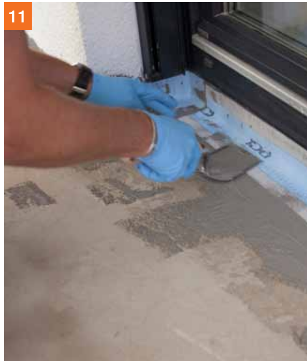
11 PCI Pectape® 120 in de PCI Seccoral® 2K Rapid bedden
