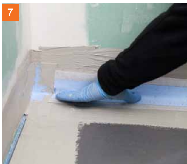
7 Breng kimband PCI Pecitape® 120 met overlap aan ...
